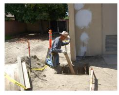
Jose Moreno, concrete finisher stamps down the concrete in the canopy footing to fill in the voids.
