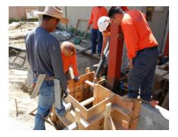
Pumping concrete into the elevator structure footing.
