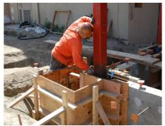
Vibrating the concrete in the elevator structure footing to help it settle and remove air voids.
