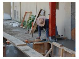
Jose Moreno trowels the concrete around the elevator structure and on top of the footings giving it a smooth surface.
